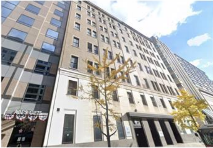
Google Maps The downtown D.C. office building at 725 13th St. NW
